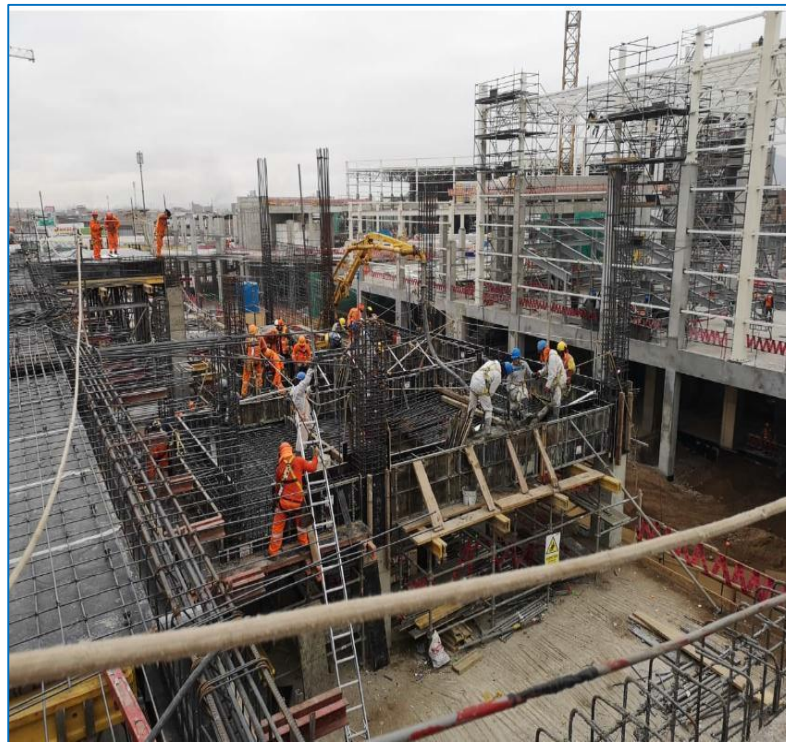
Concreto en losa – Mezzanine +8.43m, Sector 2C
