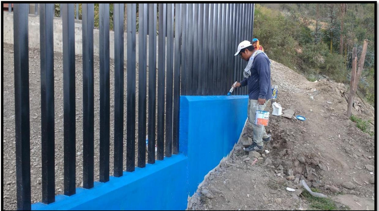
**SE OBSERVA EN LA IMAGEN NRO. 24 TRABAJOS DE PINTURA CON ESMALTE SINTENTICO COLOR AZUL NAVAL EN LOS SOBRECIMIENTOS DEL CERCO PERIMETRICO.**
