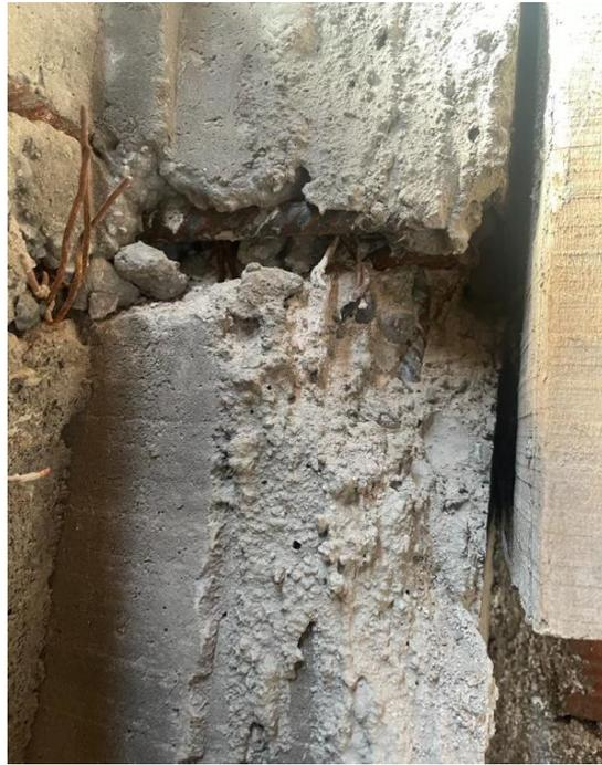
OBSERVAMOS EN LA COLUMNA PARTE DE UNA CANGREJERA A CAUSA DE UN MAL VACEADO Y ENCOFRADO
